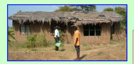
We have tried to discover why this poor thatching is the standard in Malawi when, in other parts of the world, people can construct thatched buildings that keep the water out and will last five to 10 years. There are two main problems; firstly, nobody knows how to thatch properly, and, secondly, the grass is very poor because of regular bush burning.
