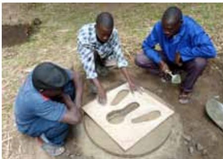
*A template is used to construct the cement cover for our RIPPLE Crapper composting toilet*
