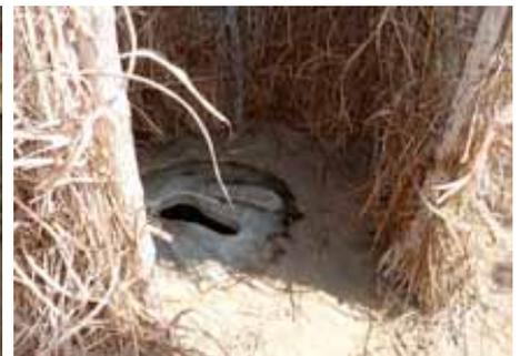
*The cement cover is placed over a circular hole to provide a composting toilet which can be used for nine months, and then the toilet is relocated*
