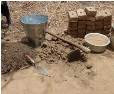
All you need is 26 bricks, a hoe, a trowel, a bucket, a 5 litre container, and clay and sandy soil
