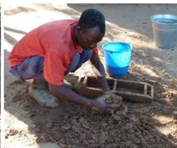
The community makes the bricks (unburnt bricks are best), either as a community or at each individual house
