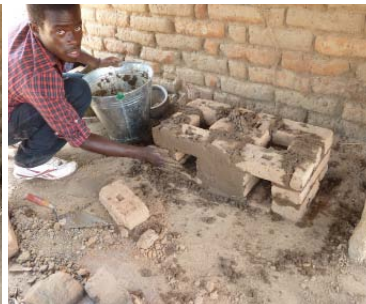
Cover the Changu Changu Moto with a mud mixture
