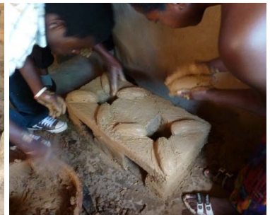
Finally, create the pot rests. The Changu Changu Moto will need regular maintenance by the householder
