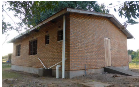
Completed ART clinic at Kande
