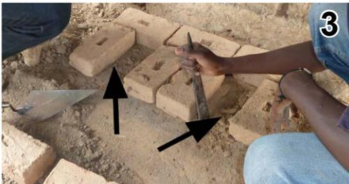
**3 Place 9 bricks in position** - Remove two bricks as shown and dig 2 holes half a brick deep (on concrete floors remove these bricks)
