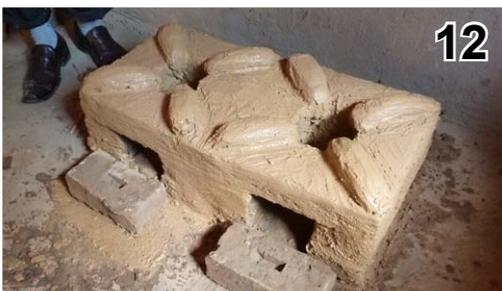
**12 Place 2 bricks outside** the fire holes - this keeps ash in the fire hole and sticks can rest on the brick. Leave the Changu Changu Moto to dry fully (2-3 days) before using
