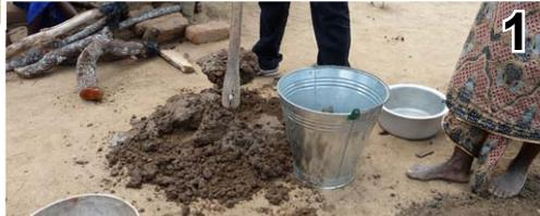
**1 Prepare mud mortar mix** - Use 5 litre cooking pot to measure soil and water. When mixed, place in bucket
