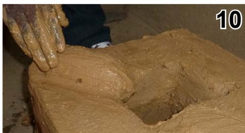
**10 Form 8 large mud pot rests** by hand and fix onto the top of the cookstove slightly overlapping the fire hole as shown above
