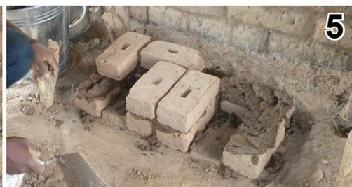
**5 Apply mud mortar mix** between and on top of the bricks, then place bricks on the next level
