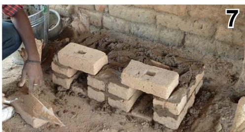
**7 Place bricks centrally over the fire holes**, then position other bricks
